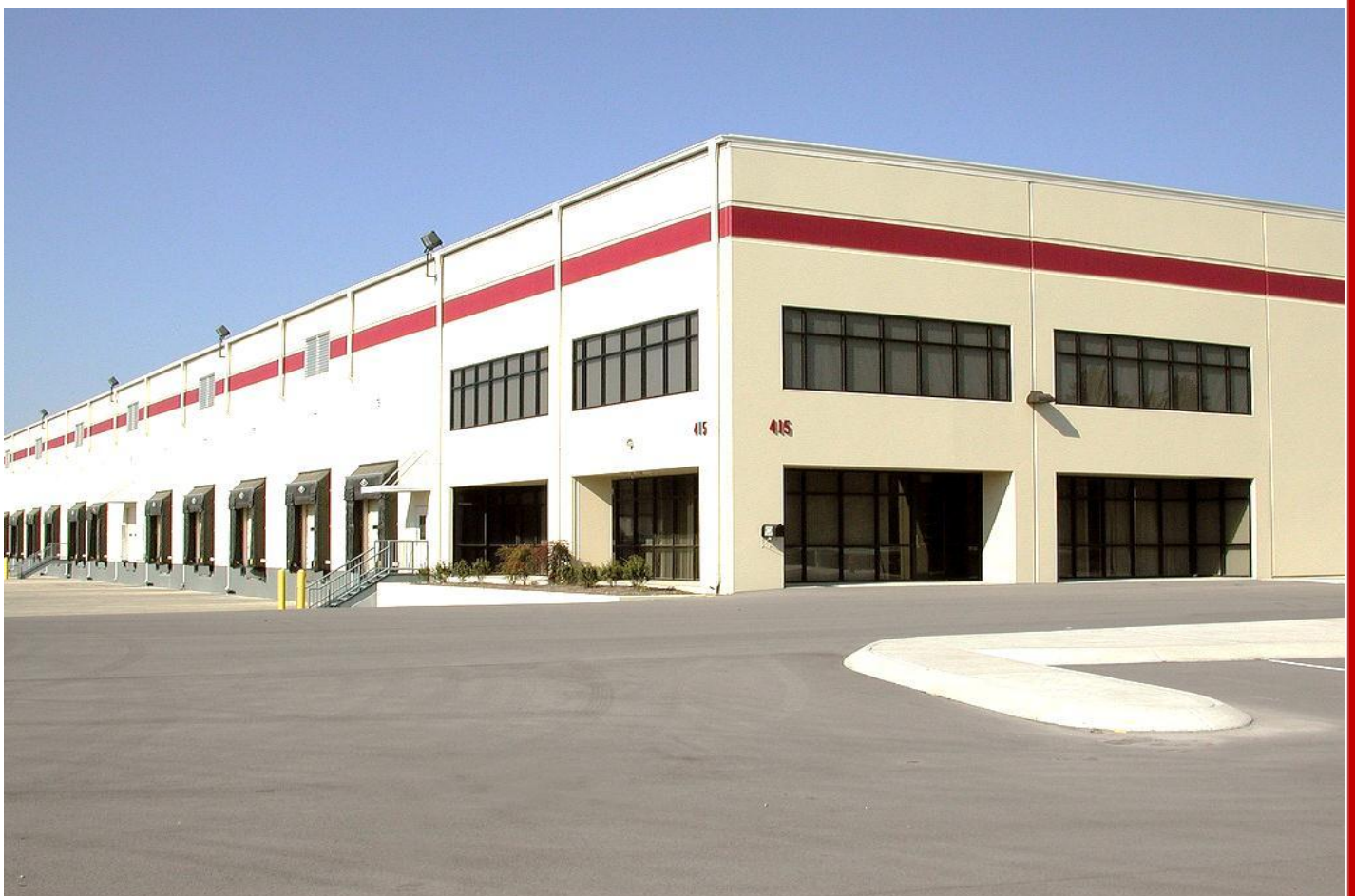
Project : G Warehouses at Hamriyah Free Zone, Sharjah Owner : Hamriyah Free Zone Authority, Sharjah
